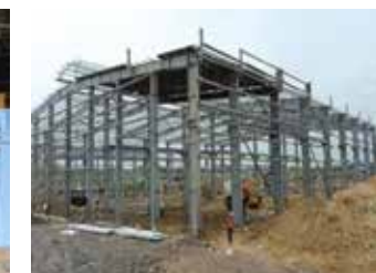
Fabricated Heavy Structure
