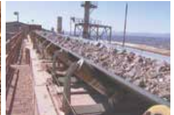
Conventional Belt Conveyor
